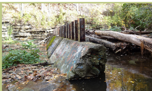
Above: Failed debris rack. If studies deem the rack eligible for removal, a maintenance plan for the MLK bridge culvert will be created.
