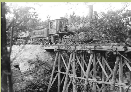
A wooden trestle built over the Doan Brook Gorge in 1915 carried trains hauling spoils excavated during construction of the Baldwin Reservoir. The fill was dumped into the Gorge. Source: Cleveland Water
