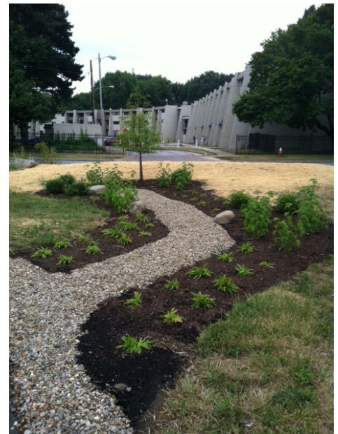
Installed rain garden at Ashbury Avenue provides improved stormwater management.
