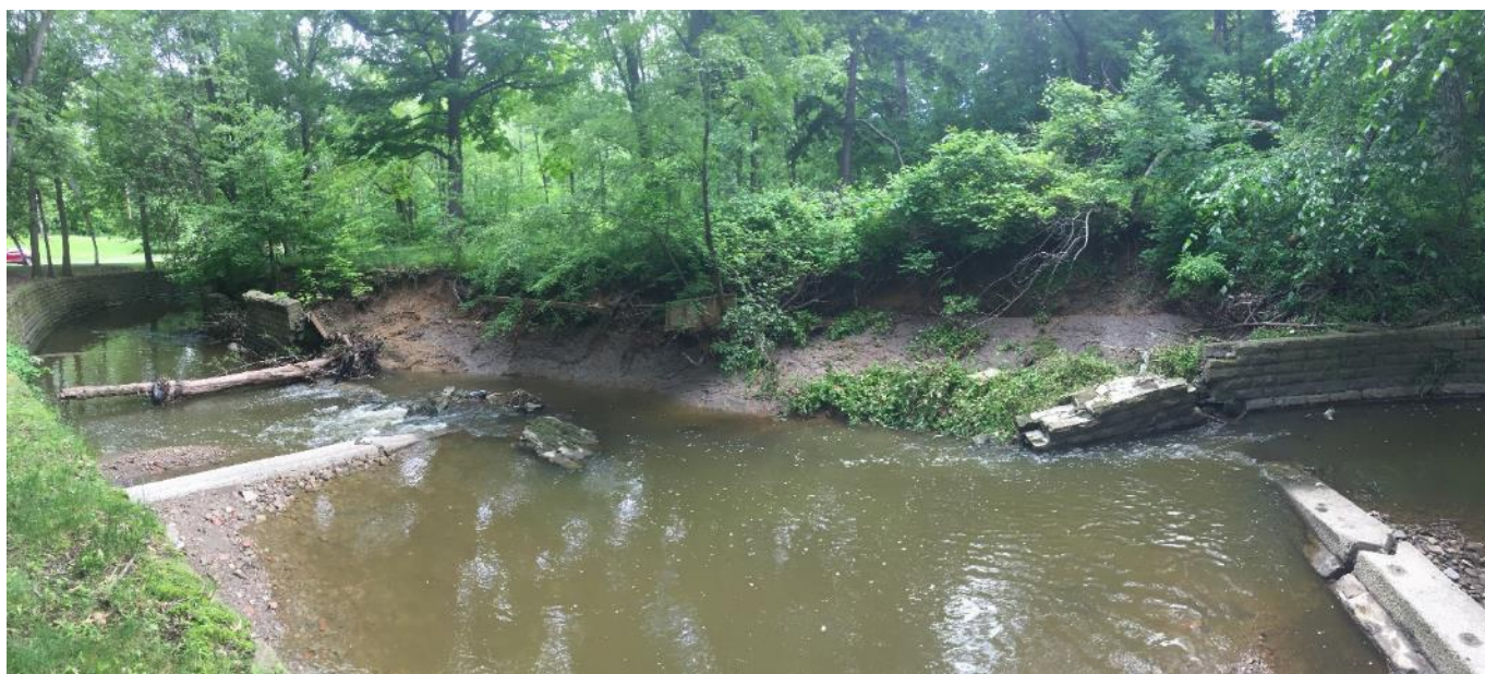
Figure 19: Doan Brook downstream of Wade Park Ave w. failing retaining walls (Photo taken June 4, 2018 by Alicia Beattie).
