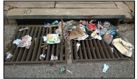
Litter ends up in our waterways when rain washes trash down the storm drain
