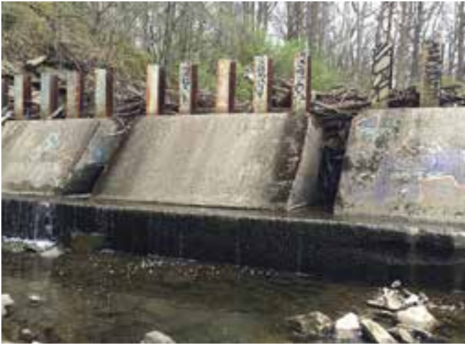
Debris rack from 1975 was removed and replaced.
